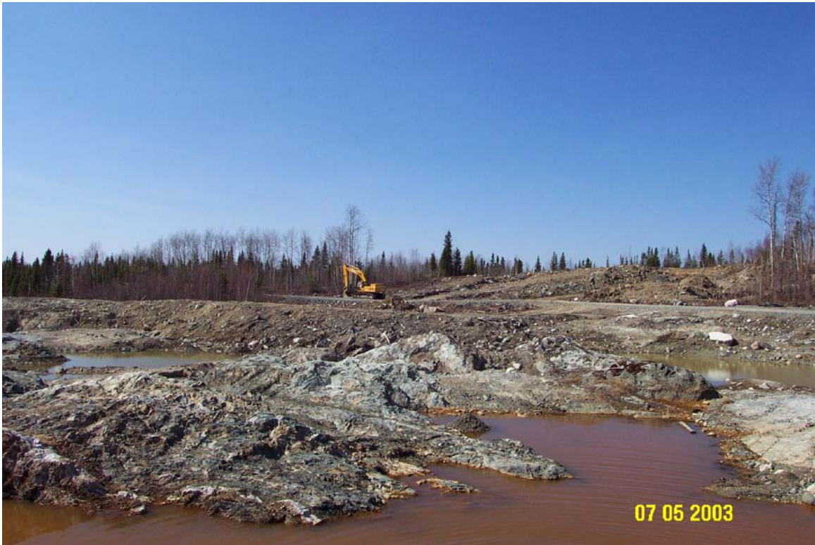
Figure 2. Surface stripping work - Dubuisson Property
