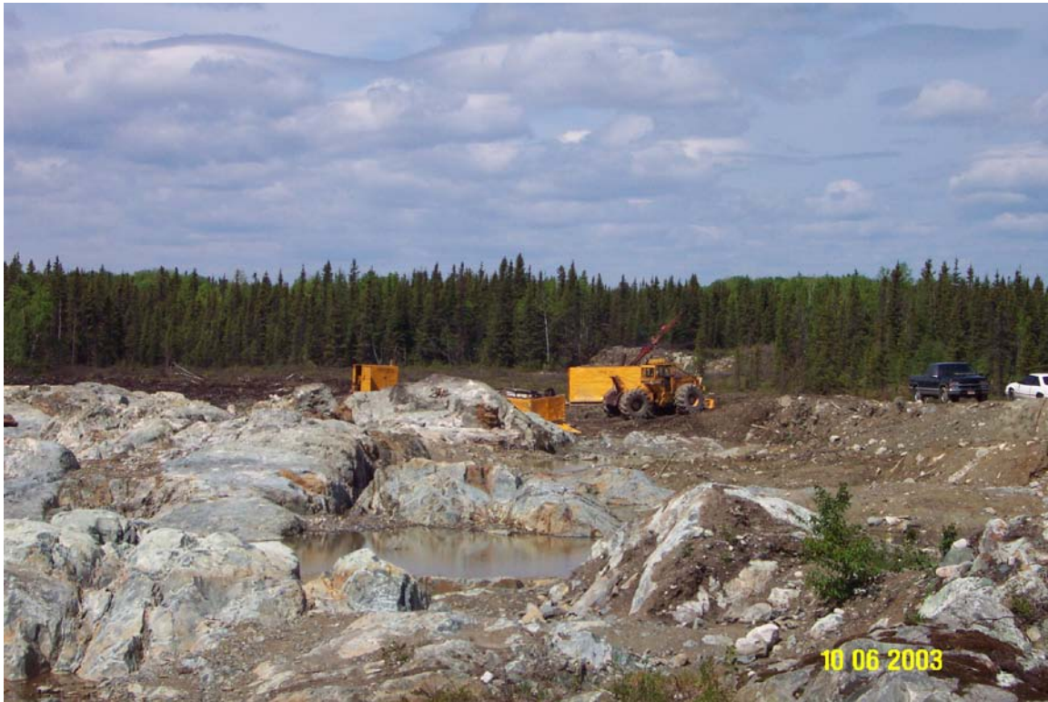
Figure 3. Surface diamond drilling – Dubuisson Property
